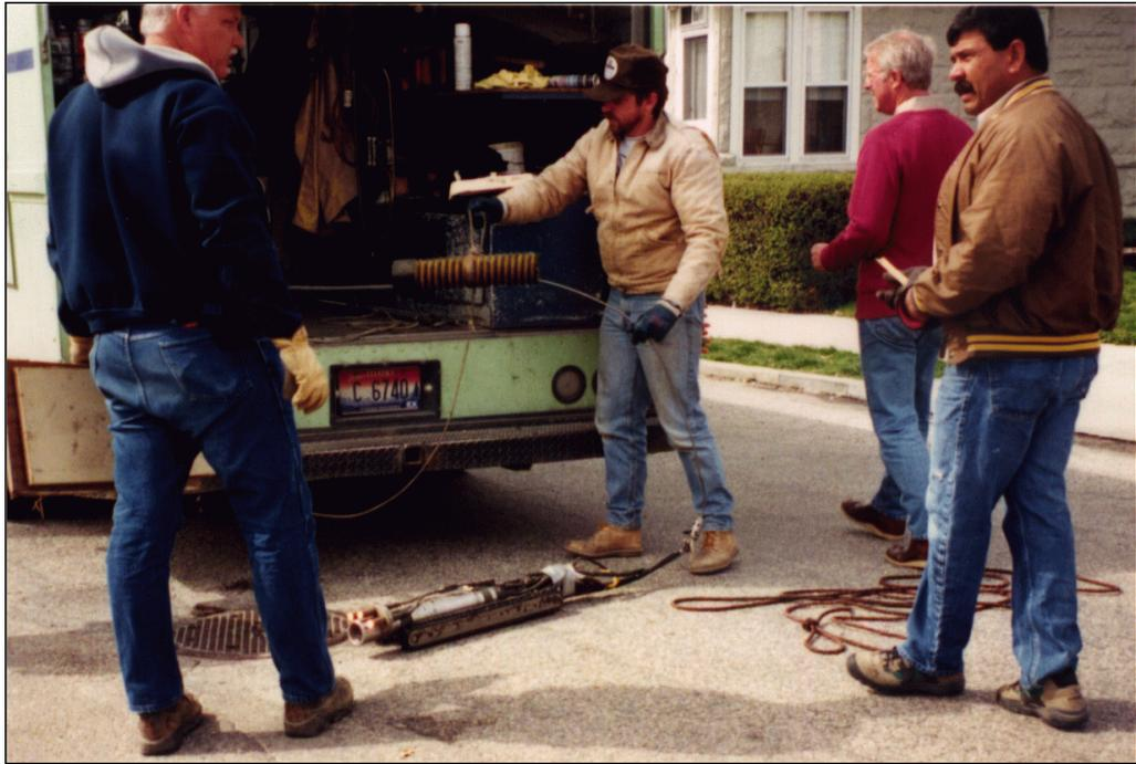
**FIGURE 5. City officials deploy a video camera to monitor the air gun's effect on a sewer line. No damage was observed in the video after multiple air gun shots were fired over a heavily cracked region of the sewer's cement wall.**
