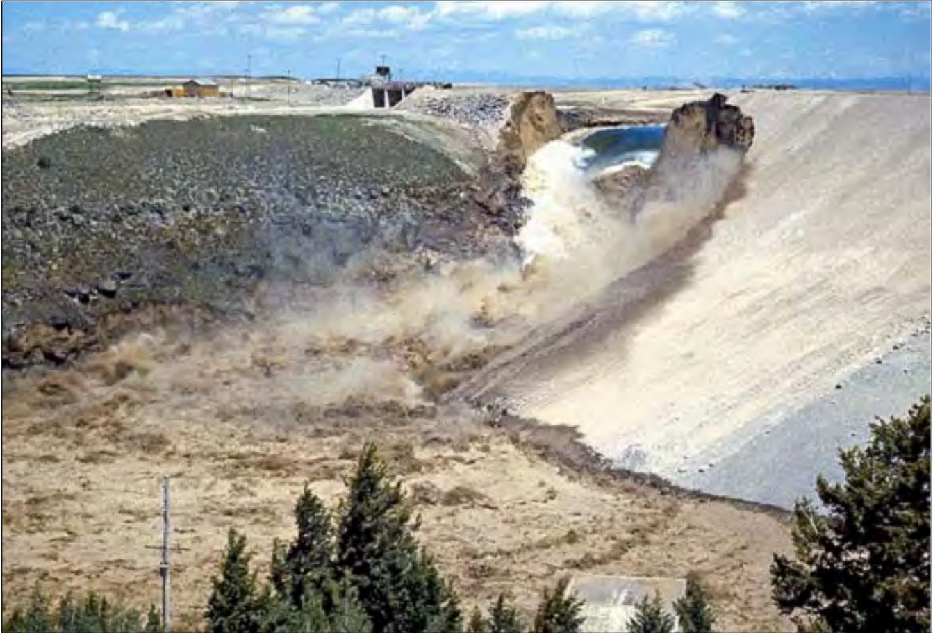
**Figure 10-1.** Teton Dam Failure, 1976
